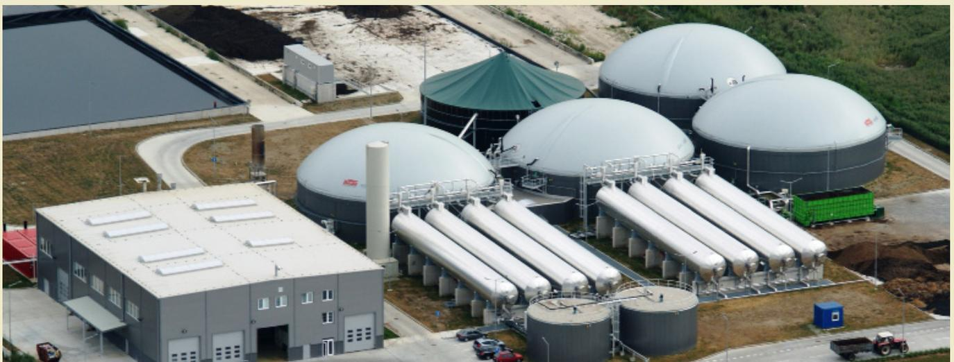
The biogas plant BOSANY is located 50km from Nitra (Slovakia). HEAT Bioenergy as a general contractor designed and built the complete plant on turn-key basis. The plant, which started its operations in 2012, is designed to process approx. 100.000 t/y of organic residues and renewables, with an electric generation capacity of 2 x 1,4 MW.
